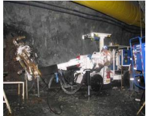
Diamond Drilling at Perseverance
