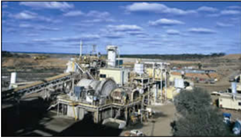
The Three Mile Hill gold processing plant
